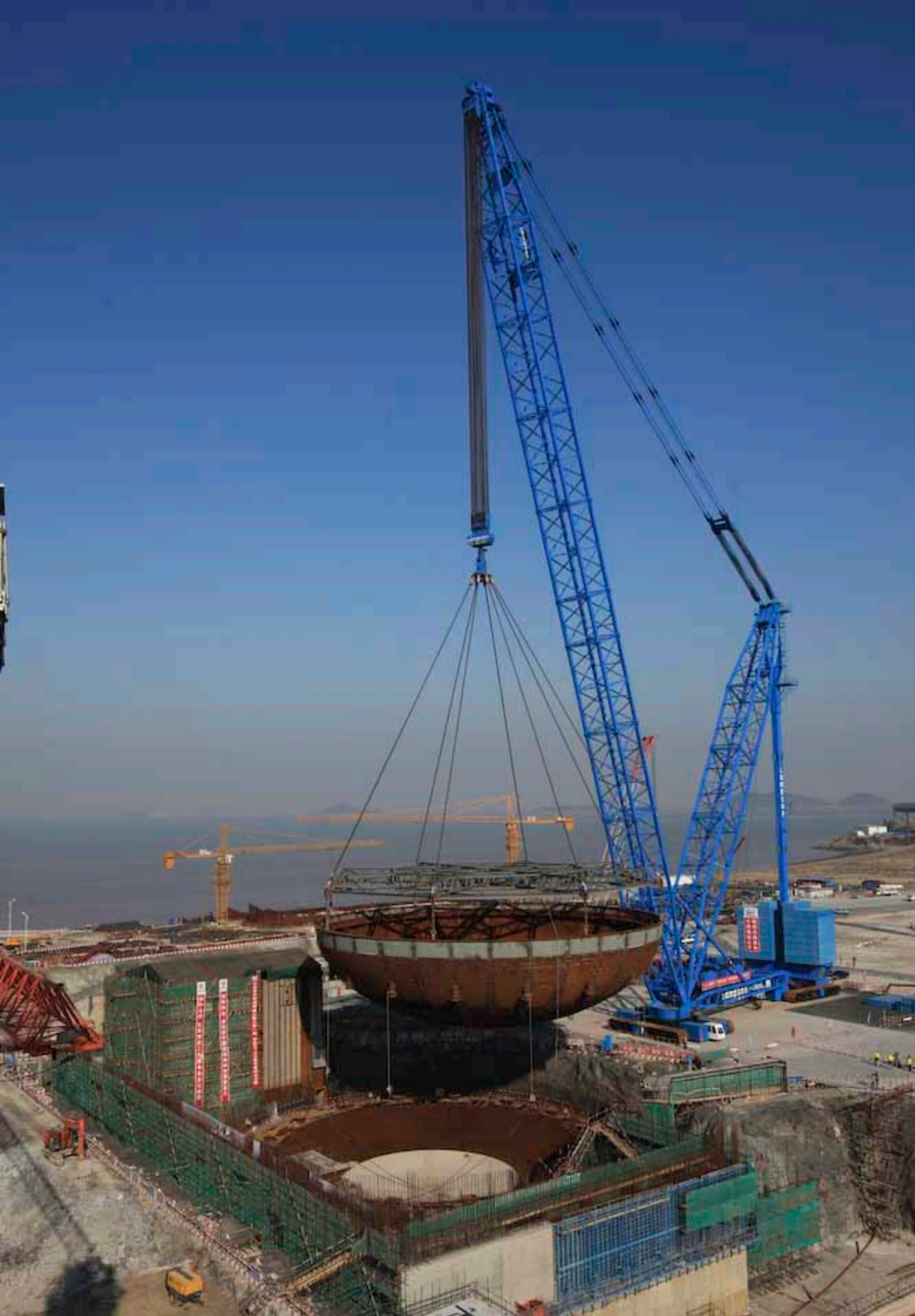
Sanmen Unit 1 - CVBH Lift
